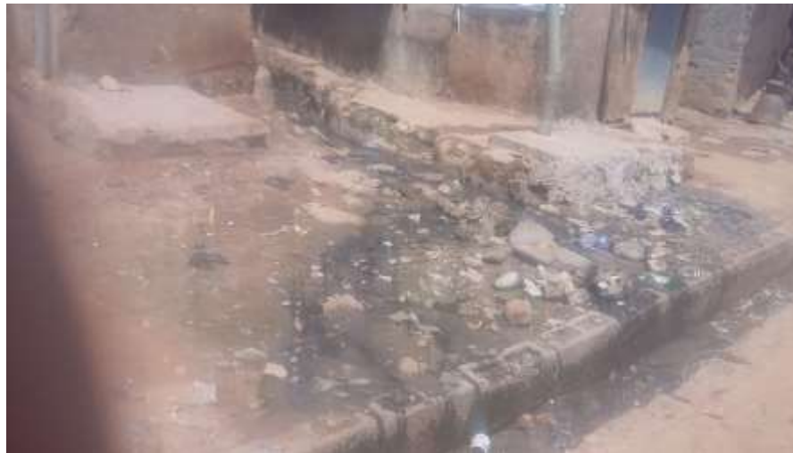
Plate 2. Open drainage. Source: Fieldwork, 2018.
